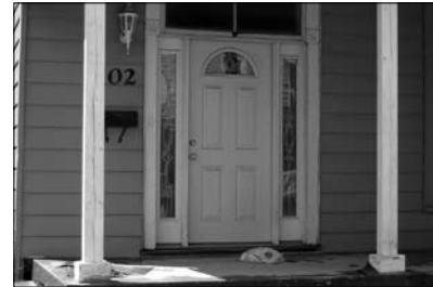
This door is not compatible with the character of the neighborhood.
