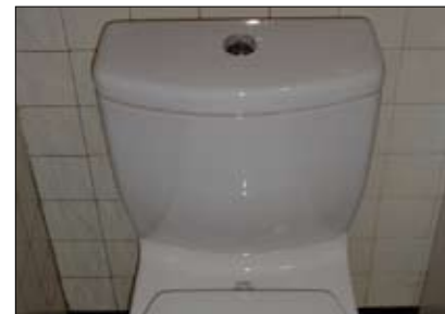
Low-flow plumbing fixtures, such as this dual-flush toilet, can reduce water use.
