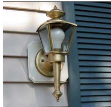
Fixtures should be durable and not made of bright shiny brass as shown.
