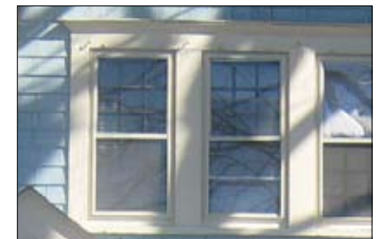
Original windows are attractive and can be made energy efficient.
