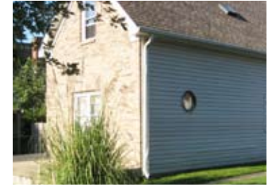
Houses that were originally made of wood siding must not be re-faced with brick.
