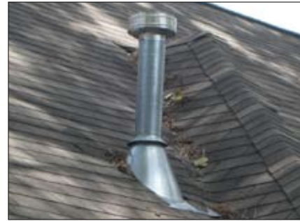
Flues should be plumb.
