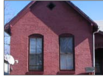
Good Existing Brick House
