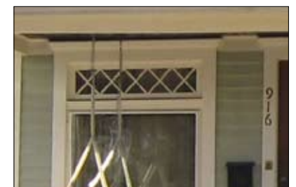
Original trim should be maintained or uncovered where possible.
