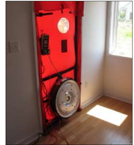
Energy Star qualified homes are tested for air-tightness. This is tested using a blower door.
