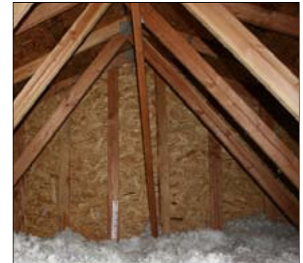
Insulation, especially in the attic, is an important energy conservation measure.
