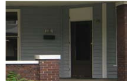
This original door opening is larger than the current door. Doors must match original openings.
