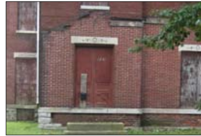
If a porch has been removed, it should be replaced.
