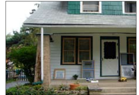
This downspout should not be placed in front of the porch column.
