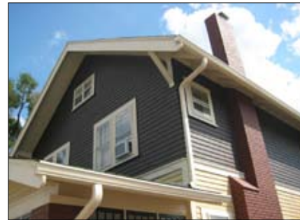
Downspouts should be placed to the sides, not at the front.
