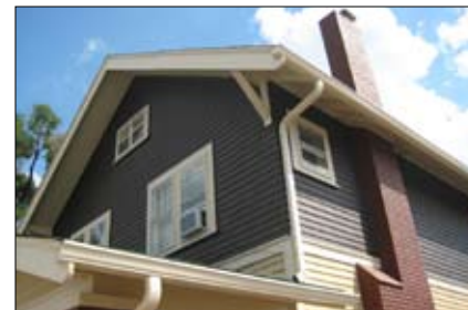
Downspouts should be placed to the sides, not at the front.
