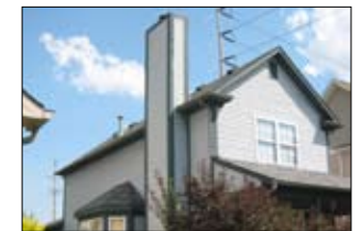
"Boxed-in" and sided exterior vertical chases that house B-vent chimneys are not permitted.
