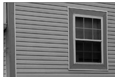
This trim is flush and offers no depth, while the siding "j" channels are too bold.
