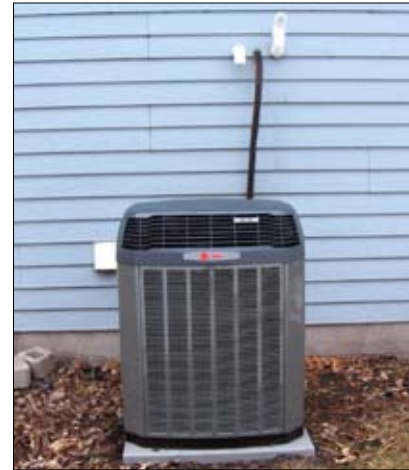
Energy Star qualified homes utilize efficient HVAC systems, like this SEER-14 air conditioner.
