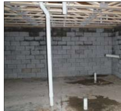
A radon system contributes to healthy indoor air. The EPA recommends radon systems for Marion County.
