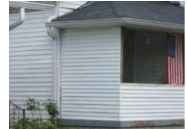
The trim on this home has been removed and replaced with very small pieces as well as covering over the porch.
