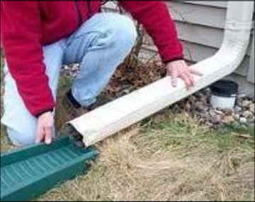
Disconnecting downspouts reduces the load on the combined sewer system.
