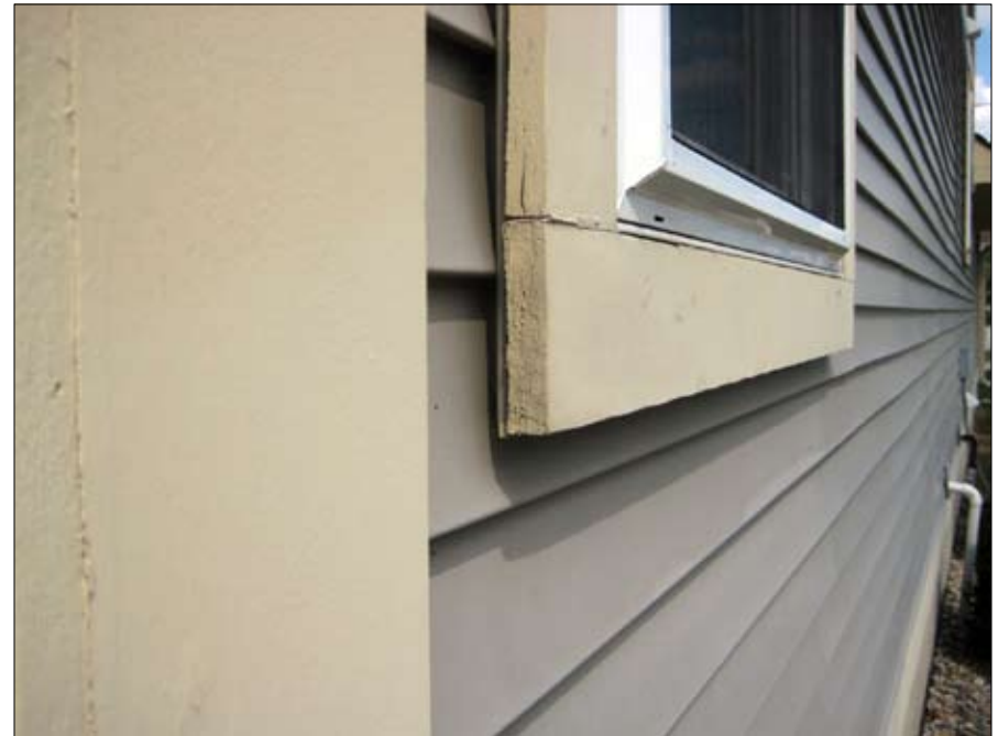
J-channels should be tucked behind trim pieces.
