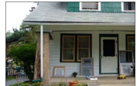
This downspout should not be placed in front of the porch column.
