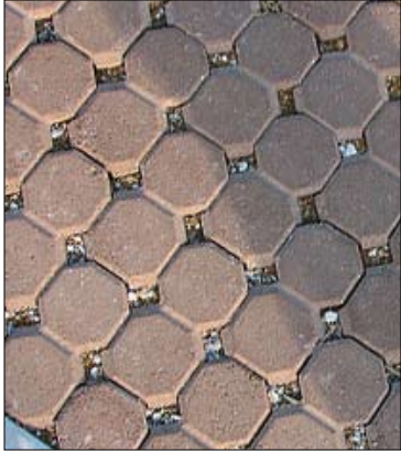
Porous paving materials help manage stormwater by reducing runoff and allowing infiltration.
