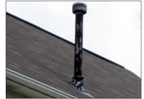
Flues should not be painted as this can later chip.
