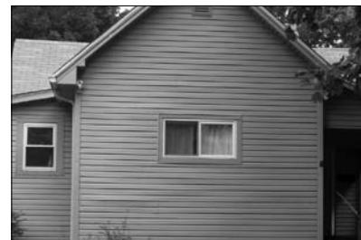
Windows should fit into the original rough openings and match existing character.
